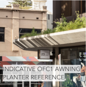
OFC1 Off-form concrete Location - Level 1 awning planters, Hotel balcony planters, Carey Street and Hotel Courtyard planter walls. External columns where indicated.
