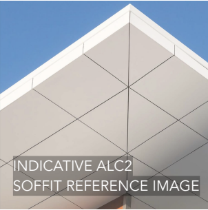
ALC 2 Pre-finished solid non-combustible aluminium cladding. Location - Colonnade and Level 1 Soffit. Residential Tower 'Skirt', 'Slots' and Parapet.
